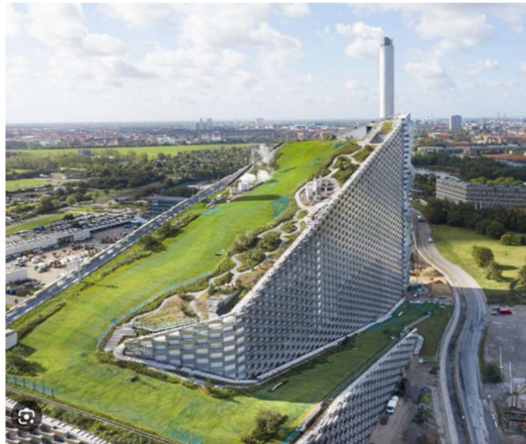
Figure 12. Amager Bakke, Co-generation plant with roof top recreational areas
